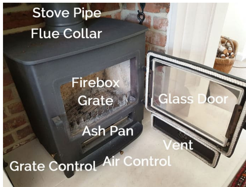
Figure 9.133. Traditional wood-burning stove components < https://fireplaceuniverse.com/parts-of-a-wood-burning-stove/ >.
